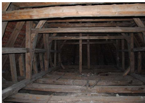
Photo 2. Truss structure with two supporting walls reinforced with dead bolts.
