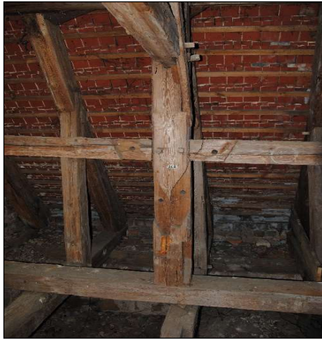
Photo 7. Places after removed struts.
