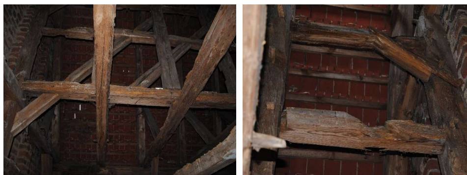
Photo 5. Bent collar beams and dead bolts
