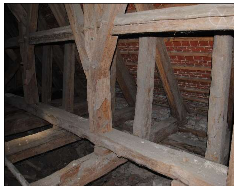
Photo 10. Wedges between the lower purlin and truss beams
